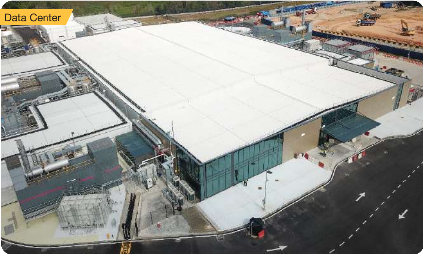
Gantry Crane Steelwork
